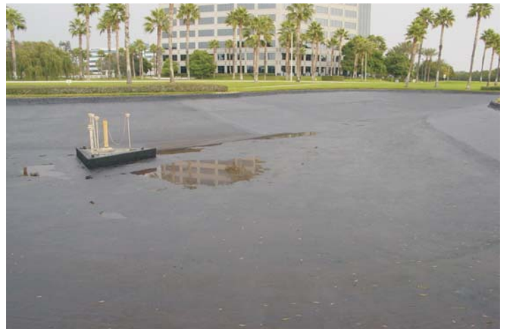
The WeatherWeld Seamless Composite system was then applied in two total passes of 30 gallons of emulsion and 16 pounds of multi-filament fiberglass roving.
