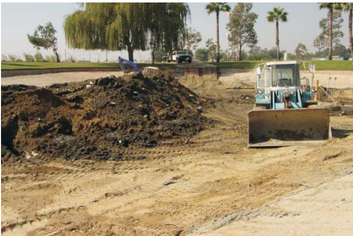
A front end bob-cat loader removed the final layers of debris and the ground was then compacted.
