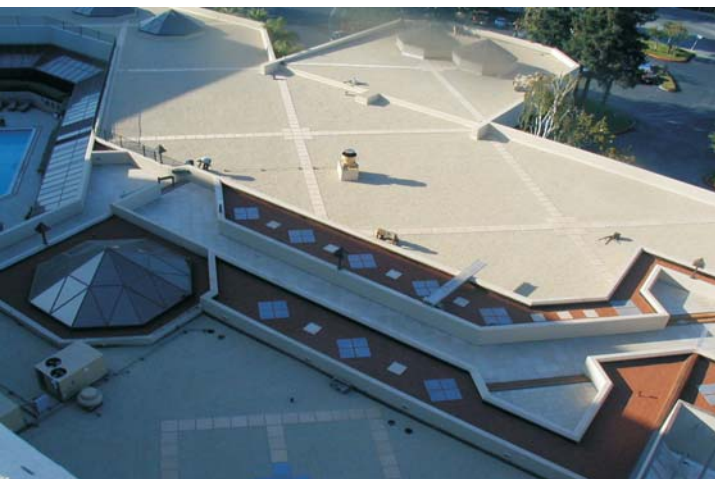
The decorative pavers were aligned to achieve the architects vision of interlocking squares, with a decorative surfacing of 3 colors of gravel, imbedded into 8 gallons of emulsion.
