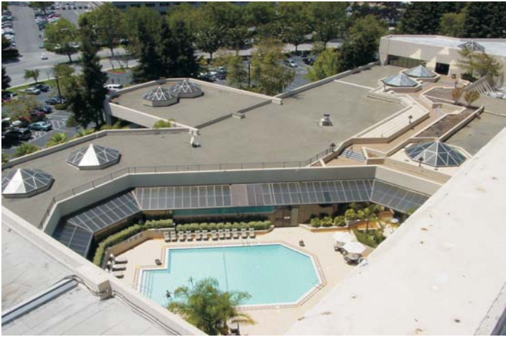
View of lower gravel roof section covering the main lobby, executive offices and hotel restaurants.
