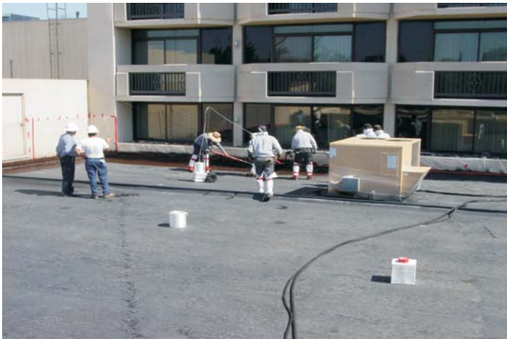
Next, two applications of the WeatherWeld Seamless Composite system were applied. The newly finished membrane would be 250 dry mils thick, with over 2.2 miles of fiberglass reinforcement per square foot.
