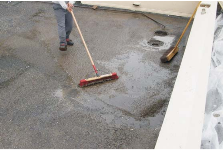
The gravel surfacing was broomed, vacuumed and broomed.
