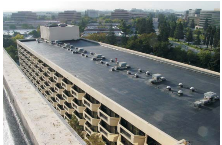
View of Southern roof the day after its 1st application.
