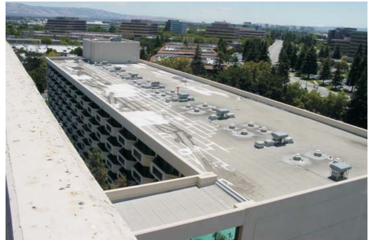
From same elevation, view of the Southern facing 8 story building.
