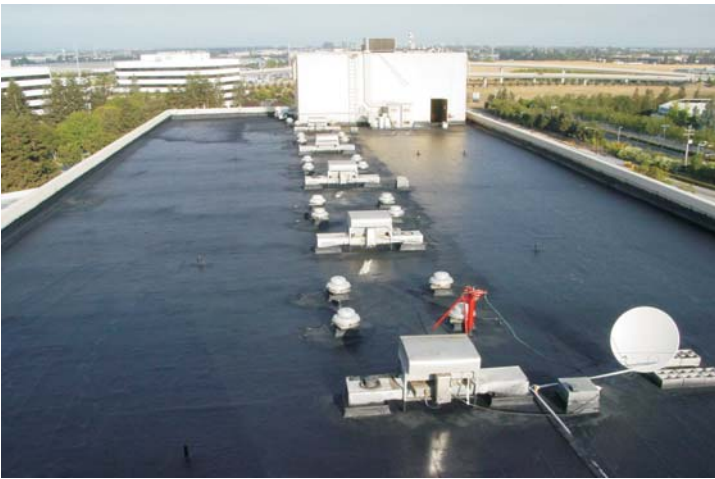
View of Northern roof after 1st pass of the WeatherWeld system.
