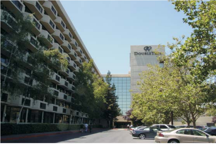
Project: reinforcement of existing roofing assembly for the DoubleTree Hotel, San Jose, California. Project specified the WeatherWeld 16-30 Seamless Roofing System.
