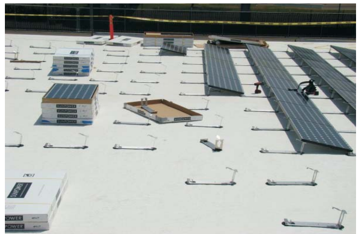
Designed for fast and easy installation, T10 solar tiles are non-penetrating and lightweight, highly durable, and resistant to high wind speeds up to 120 mph (193 km/h).
