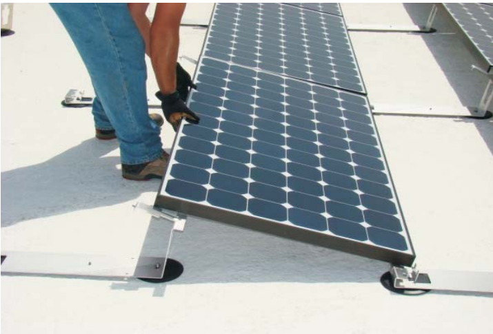
The SunPower T10 Solar Roof Tile tilts at a 10-degree angle to increase energy capture.
