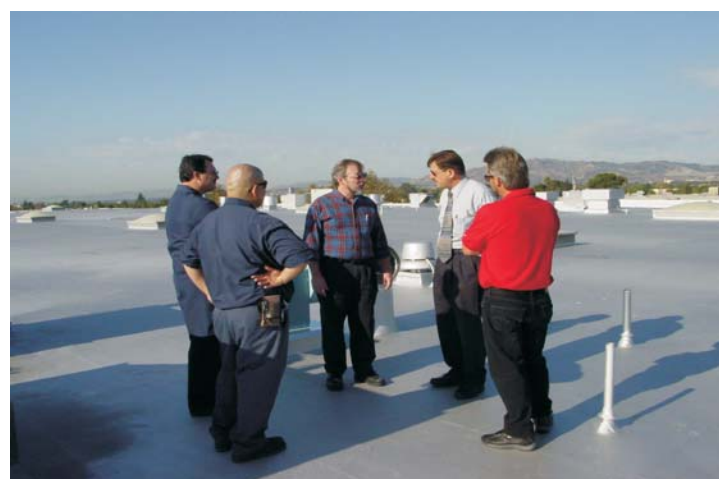
At the final job walk, three members of the facility's management team, the contractor and the property management company's consultant enjoy the results. For your company's piece of mind, call us at 888-440-3224.
