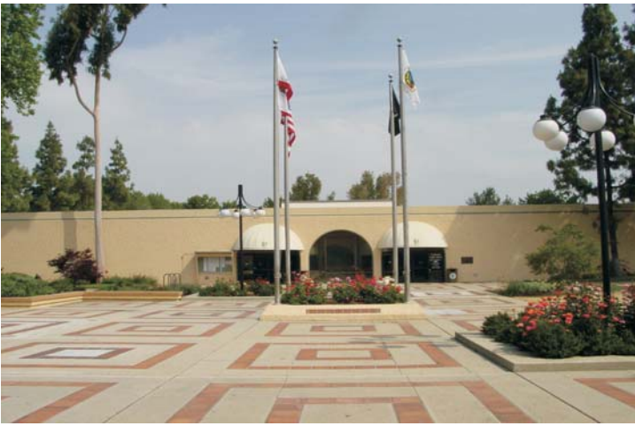
View of main entrance of City Hall.
