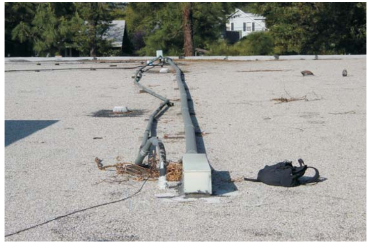
Assembly is metal deck, covered with light-weight concrete, covered with 1" fiberboard insulation, covered with a 4 ply BUR set in hot asphalt, cover with a gravel surfacing.
