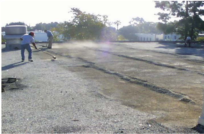
Gravel surfacing is vacuumed, broom and vacuumed.
