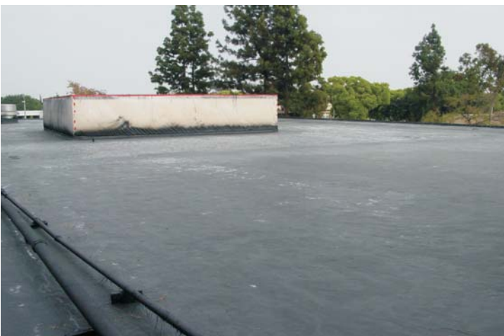
A double pass of WeatherWeld seamless composite is applied.
