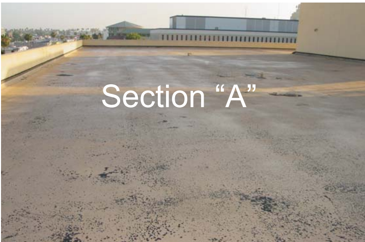
Section "A" has been power washed in preparation for its application.
