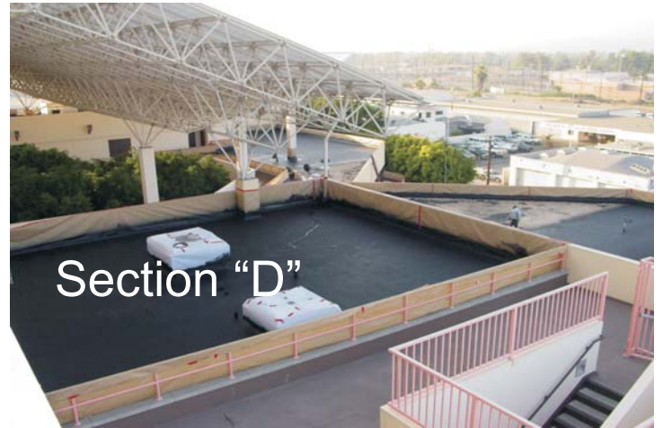
Completed Section "D" overlooking lower Section "H".
