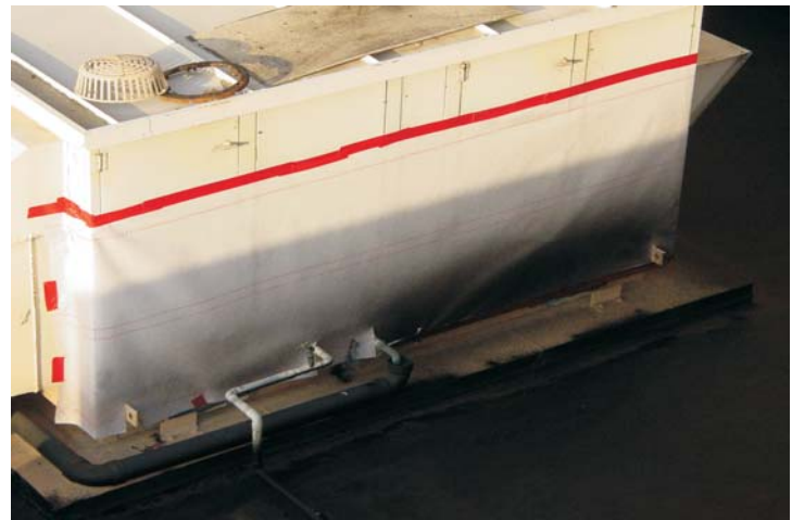
To ensure an uninterrupted flow of air to the A/C units, they were masked-off using polyester.
