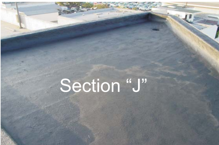
Completed Section "J" on the SE corner of structure.
