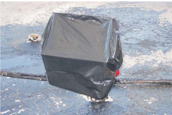
Flood lights were covered with polypropylene to protect them from over-spray.
