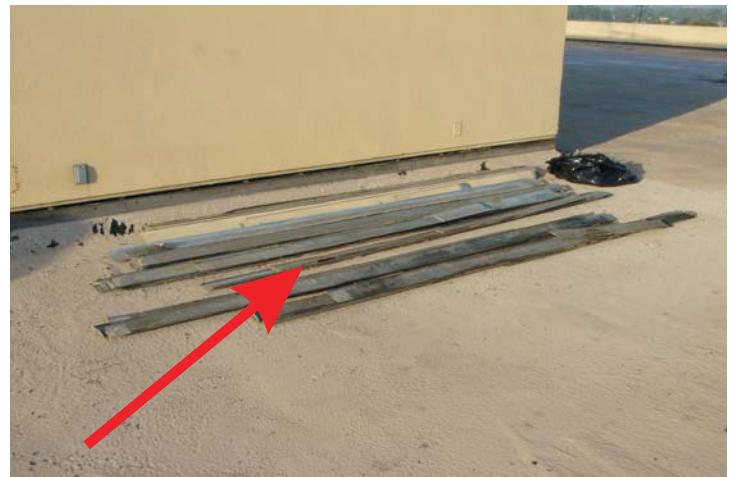
The metal counterflashings have been temporarily removed to apply the seamless composite up to the reglet above the baseflashings. These counterflashings will then be reattached.
