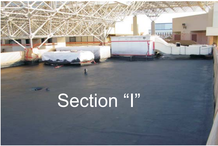
View of the first pass of WeatherWeld on Section "I".
