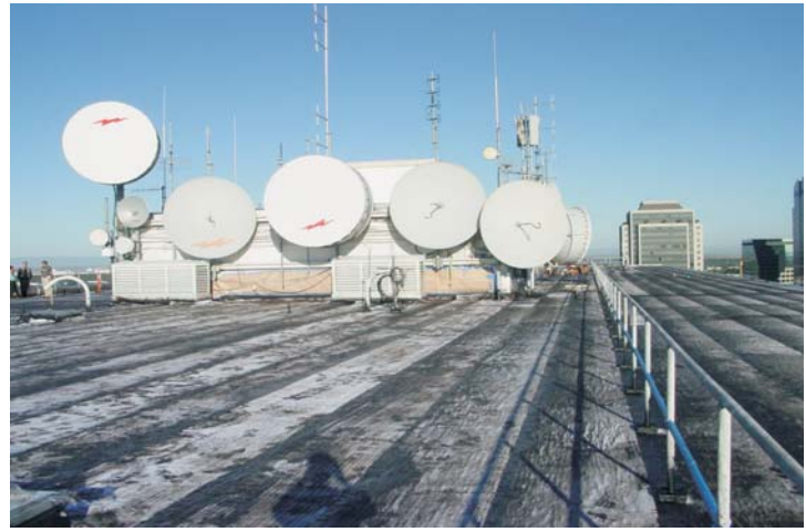
View of the polyester scrim as it cures out in the sun.
